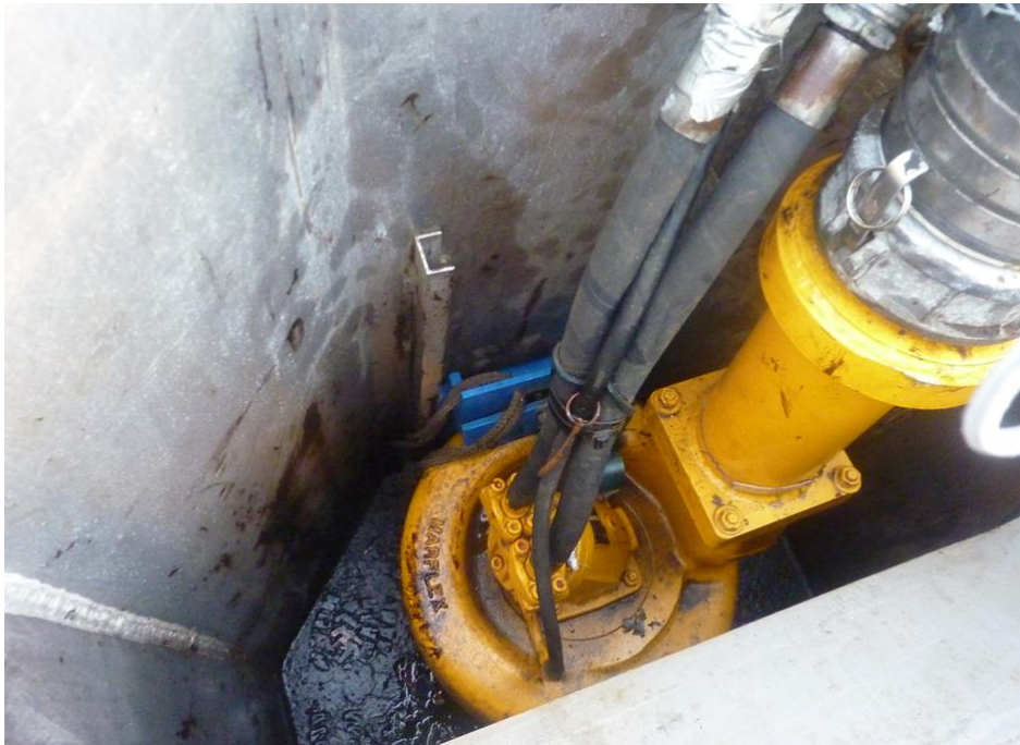
Figure 7 MSP 150 installed in the weir skimmer module
