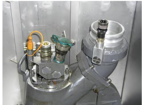
Figure 9 Lamor water injection flange mounted on a GTA pump
